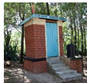
Trisan toilet with twin sets, where urine and composted feces are both used in agriculture
